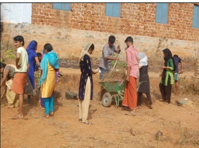
School Playground Construction (12 May 2019, 13 May 2019)
