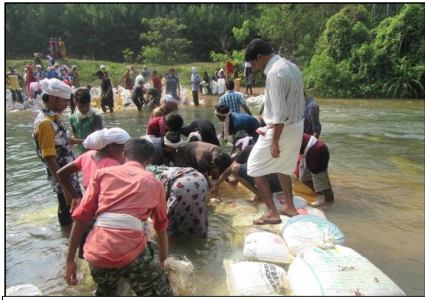
Construction of Bund-ATHIJEEVANAM (10 February2020,11 February 2020)
