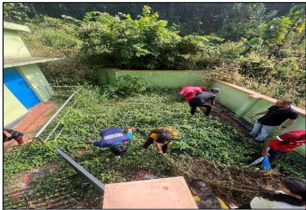
Take a Break Restoration Programme - Renovation Programme in Karakurussi Panchayath (25 December 2023)
