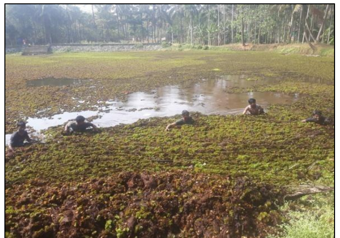
Perumkulam Renovation (May 2019)
